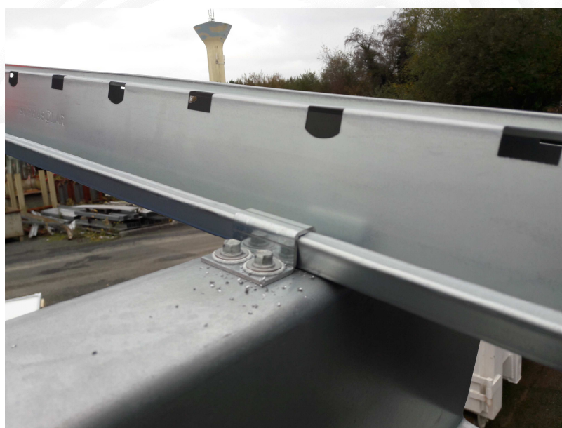
IMPLEMENTATION OF THE SOPRASOLAR CRAPAUD
